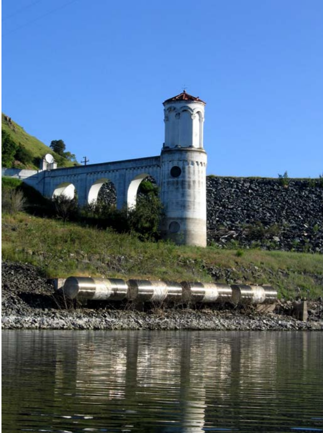
Figure 1-1. Calaveras Dam adit structure and exposed upper adit.
